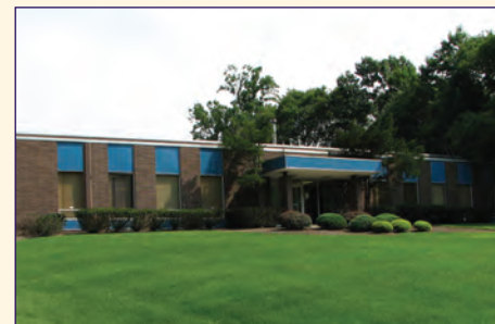
Avtron Industrial Automation, Inc., Digital Facility, Independence, Ohio.
